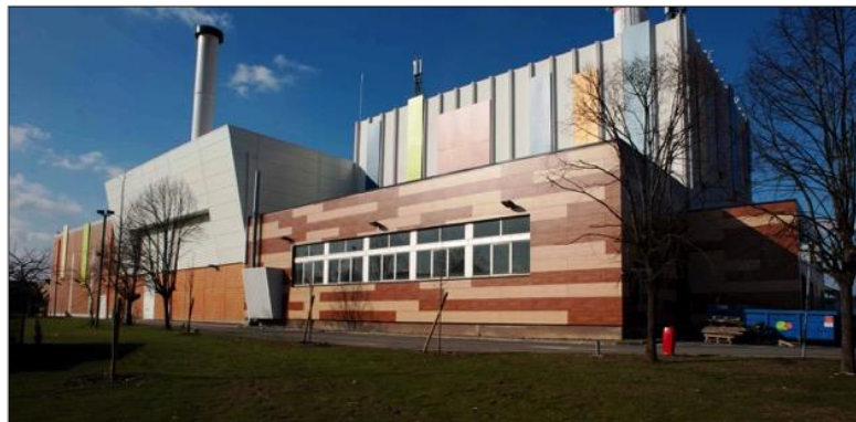
Photo Chauffage Stains - Aline Bros
