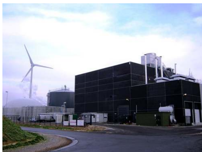
Installation BIOTIM® Wet AD, Belgique
